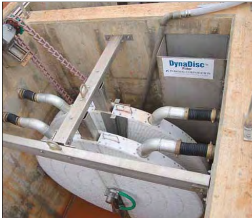
Figure 4.5 DynaDisc ® Cloth Media Filter
