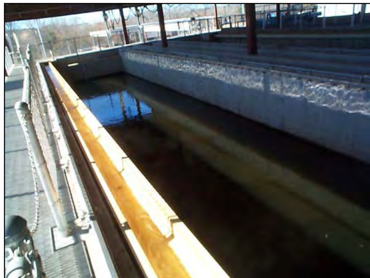
Figure 4.2 Typical Filter Bed
