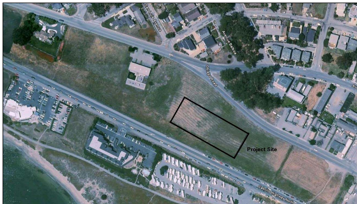
Figure 3 Project Construction Site
