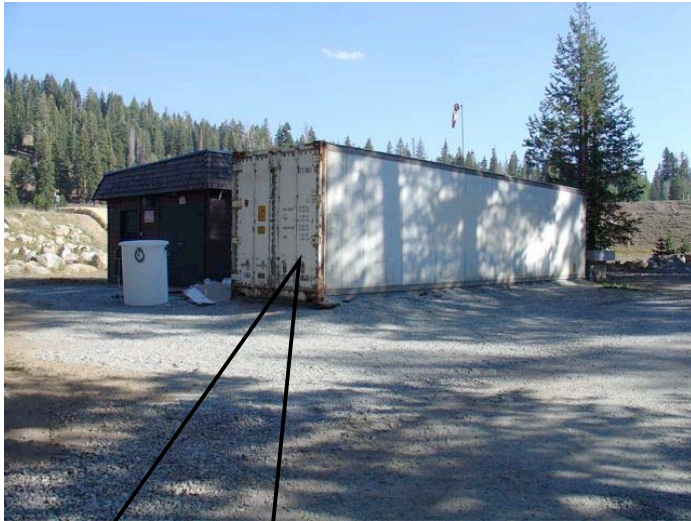
Exterior: Insulated Container (Fall)
