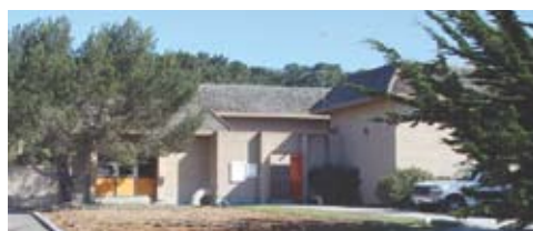
The Portola pump station in El Granada.
